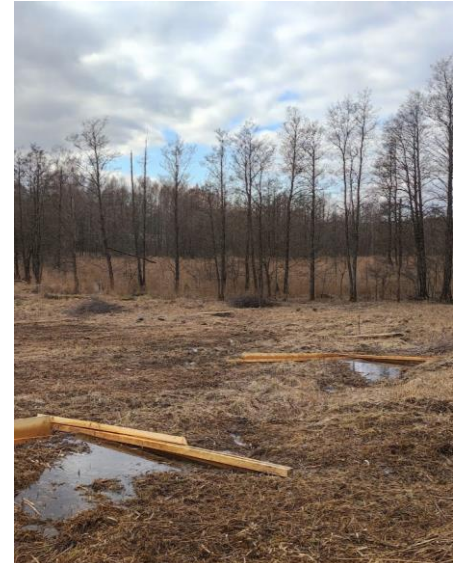
Dams of various constructions were installed on drainage ditches.
